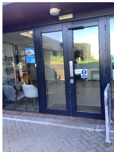
Church Hall Lobby Entrance
