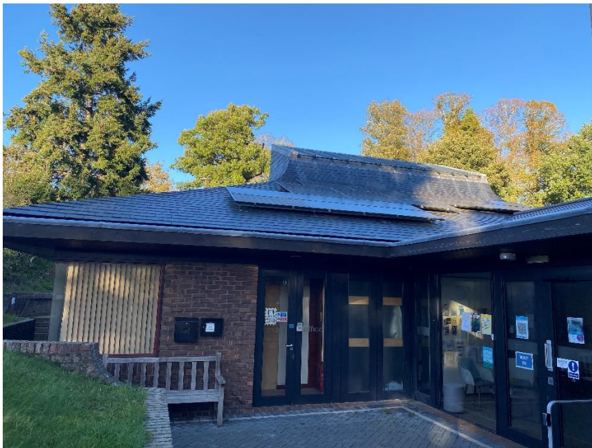
Photo of existing PV installation taken at 3pm on 1 November 2021.
